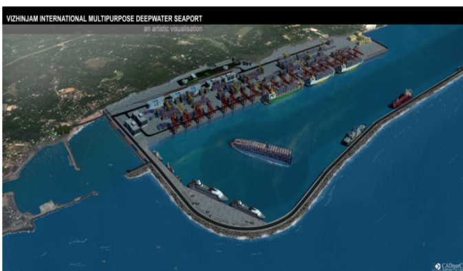
Vizhinjam international multipurpose deepwater seaport
