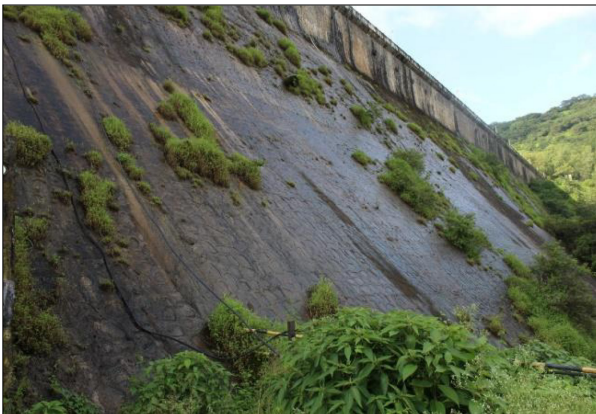
Downstream view of Warna dam at FRL before partial grouting
