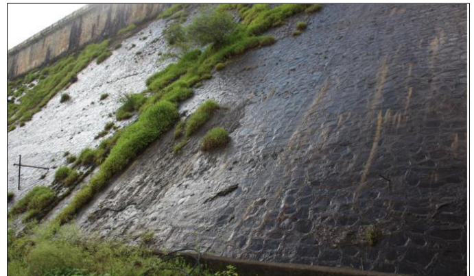
Downstream view of Warna dam at FRL before partial grouting
