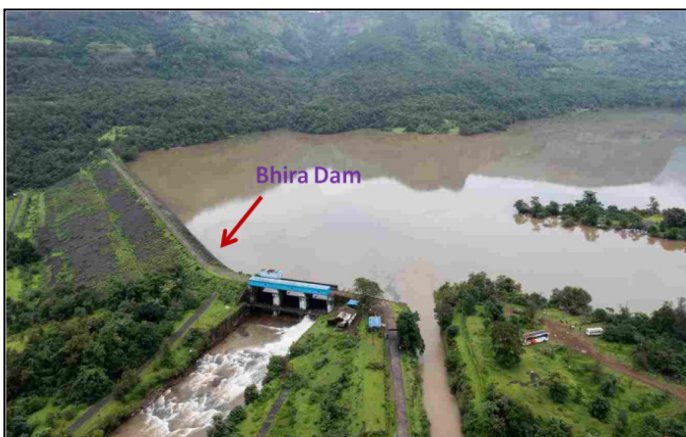
Aerial view of Bhira Tailrace Dam, Maharashtra
