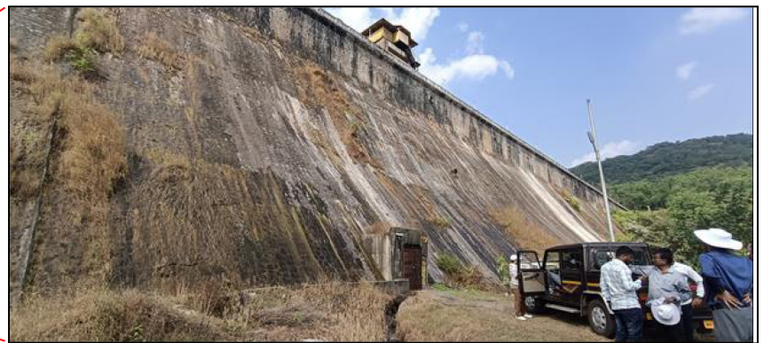
Downstream view of Warna Dam at FRL at Partial Post Grouting Stage
