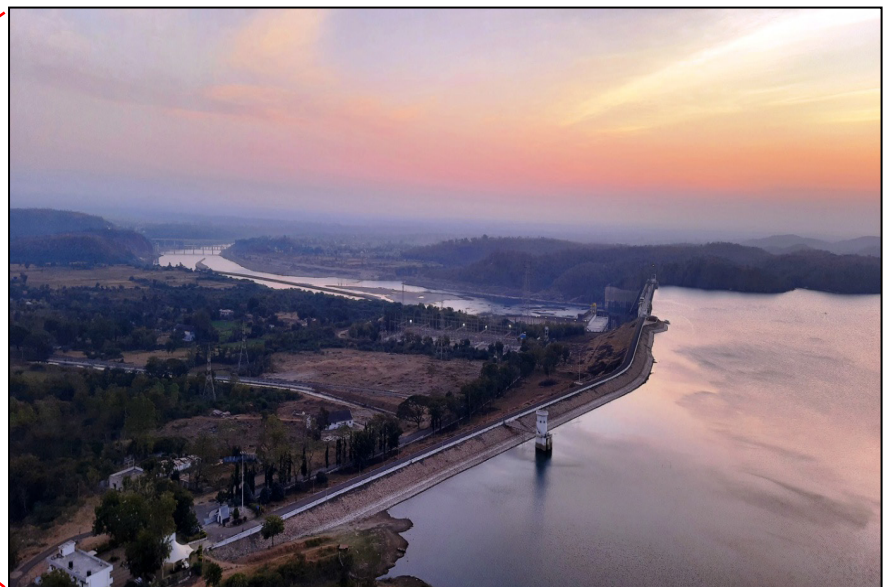
Panoramic view of Kadana Dam, Gujarat
