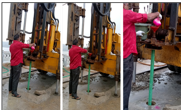
Tracer Injection in 150 mm borehole
