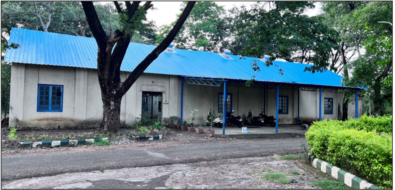
Ingress protection laboratory at CWPRS, Pune
